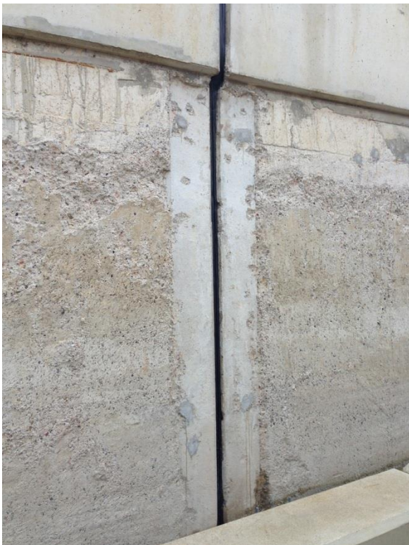
Prefab betonnen dilatatiebalk in diepwand dive-under
